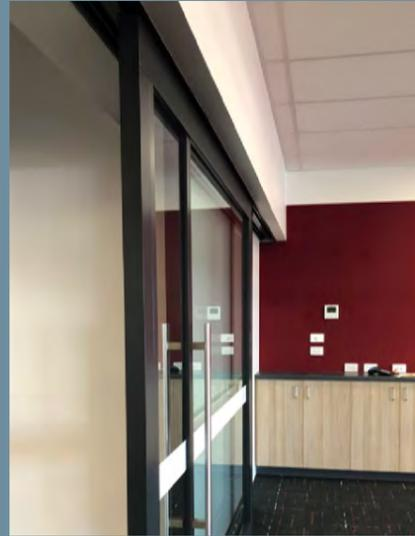
Easily access Classique sliders for servicing. The tracks can be fully recessed into the ceiling or bulkheads, as there is no need for ceiling access after they are installed.
